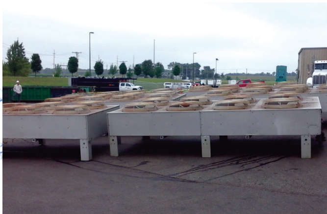
NIMBUS replaced these seven 8-fan dry air coolers with two 5-fan VIRGA III systems.
